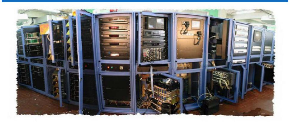
All necessary components are concentrated into few modular cabinets. With previous conventional equipment, components were distributed in various locations on the ship.
