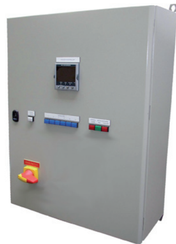
Electric heater control cabinet
